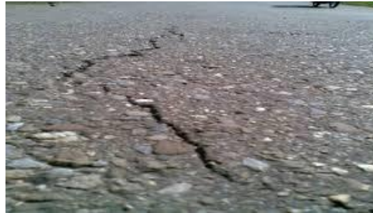
Gambar 3.20 Pelapukan dan butiran lepas ( weathering and raveling ) Sumber : Bina Marga No.03/MN/B/1983
