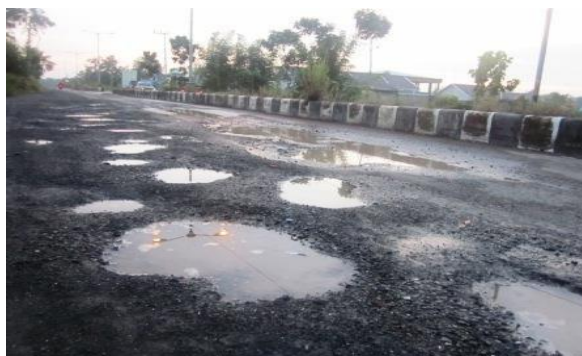
Gambar 3.25 Lubang ( Potholes )
