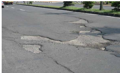
Gambar 3.23 Pengelupasan ( Delemination )
