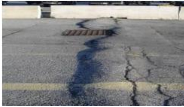
Gambar 3.10 Benjol dan Turun ( bump and sags ) Sumber : Bina Marga No. 03/MN/B/1983
