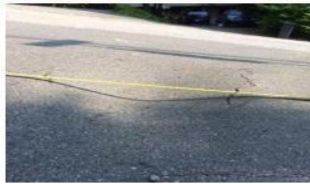
Gambar 3.7 Amblas ( Depression ) Sumber : Bina Marga No. 03/MN/B/1983
