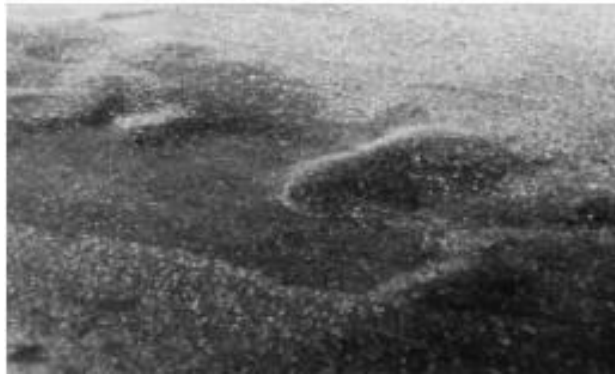
Gambar 3.8 Sungkur ( Shoving ) Sumber : Bina Marga No. 03/MN/B/1983
