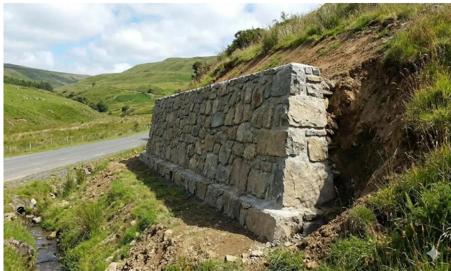
Gambar 3.1 Dinding Penahan Tanah Gravitasi
