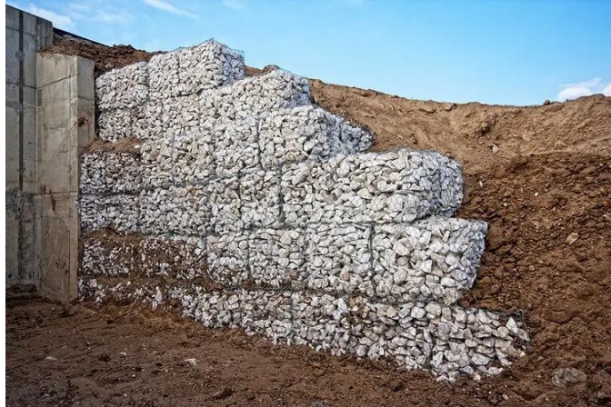
Gambar 3.4 Dinding Penahan Tanah Bronjong
