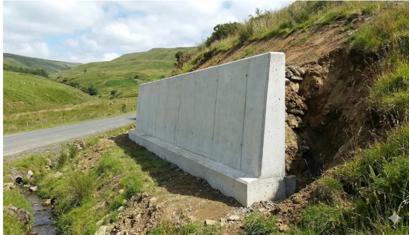
Gambar 3.2 Dinding Penahan Tanah Kantilever
