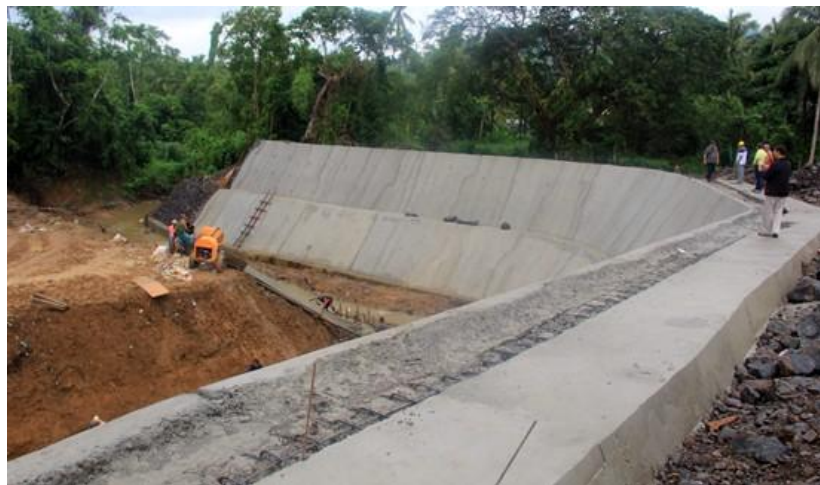
Gambar 3.3 Dinding Penahan Tanah Bertulang
