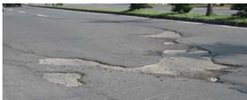
Gambar 3. 24 Pengelupasan ( Delemination )
