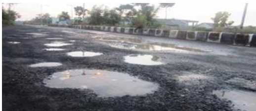
Gambar 3. 26 Lubang ( Potholes )
