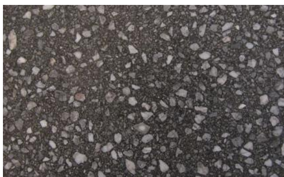
Gambar 3. 9 Kerusakan Polished Aggregate
