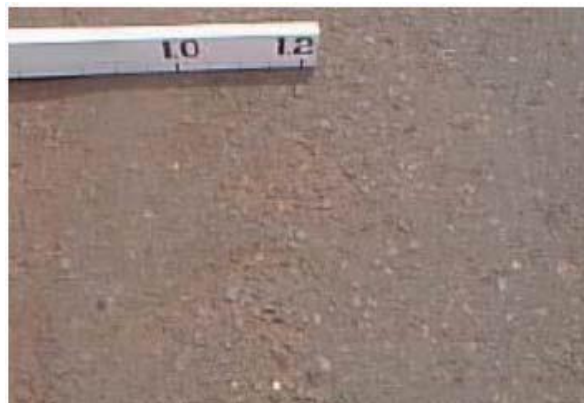
Gambar 3. 13. Pengausan Agregat ( Polised Agregat ) Sumber : Bina marga no.03/MN/B/1983
