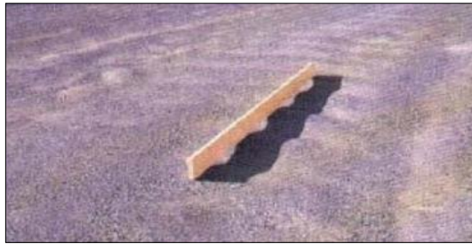
Gambar 3. 6. Keriting ( Corrugation ) Sumber : Bina marga no.03/MN/B/1983
