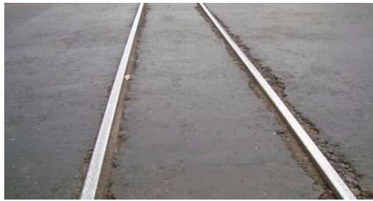
Gambar 3. 15. Rusak Perpotongan Rel ( Railroad Crossing ) Sumber : Bina marga no.03/MN/B/1983
